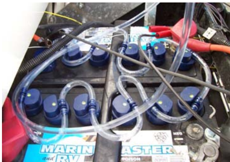
(AquaPro Fill-cap installed on Deka battery)
